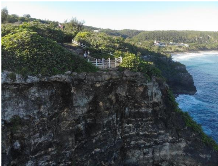
FIGURE 1: STUDY AREA IN QUEBRADILLAS, PUERTO RICO
